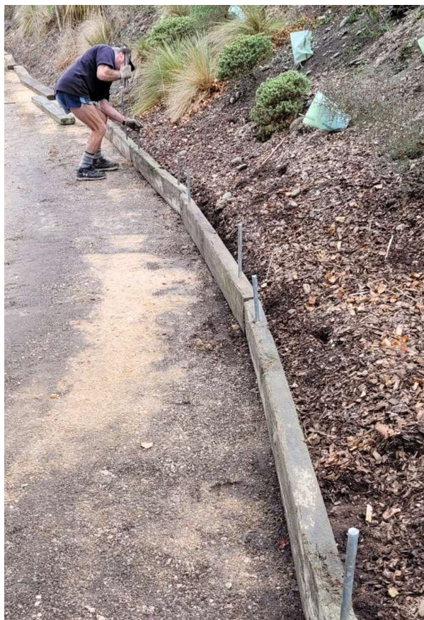
Lloyd Grafton installing the timber edging
